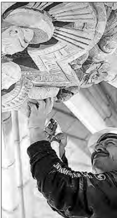
Phase I repairs began in March 2014 and addressed the interior high ceiling of the nave and restoration of the six flying buttresses around the apse, or east end of the Cathedral.
