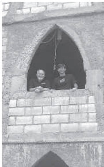
Father Paul Martin and Mickey Quinlan look out over the village from an upper level of the newly roofed church.
