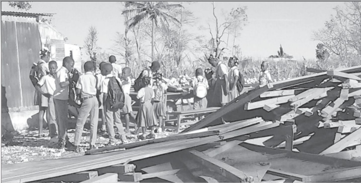
Students at the Episcopal primary and secondary school in Bégin, Haiti survey the damage done to the kindergarten building during the passage of Hurricane Matthew.
